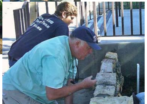
Constructing several planter boxes out of stone and mortar (right) was also part of the project.
